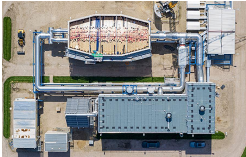
Figure 26: Packed-Bed sensible storage with rocks. © Copyright: Siemens Gamesa Renewable Energy / Ulrich Wirrwa., Image taken from [76].
